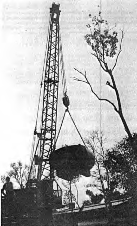
BIG LIFT -- Relocation of the 4th Division's base camp necessitated the installation of several additional water tanks at Camp Radcliff.
